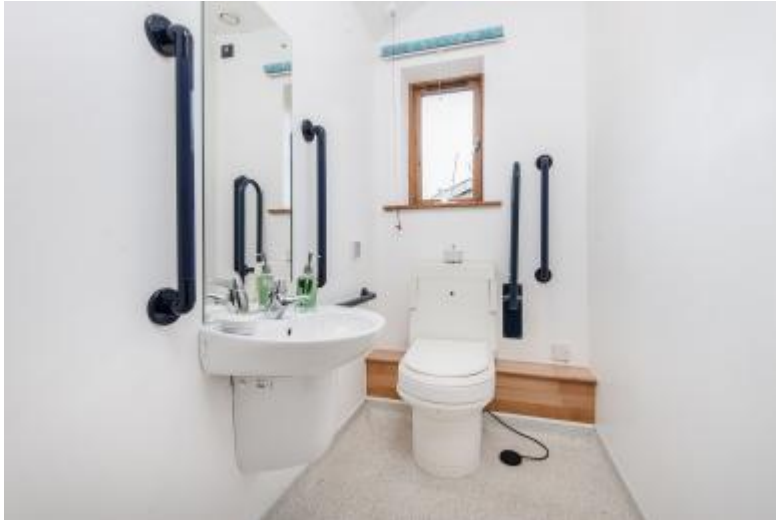
Downstairs cloakroom with Close-O-Matt shower w.c. Wash basin with lever taps front transfer
