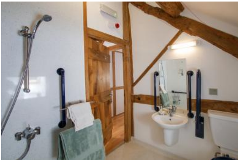
Wet-room , Altro non-slip floor, contrasting fixtures , emergency lighting.
